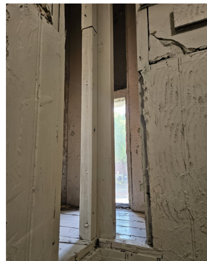
Current state of bathrooms
