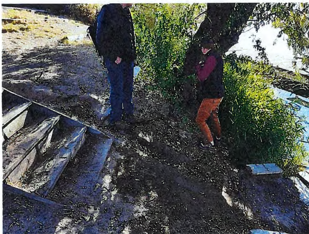
Figure 2: Erosion gullies can be seen extending from parking lot elevation down to the water surface; additional damage is visible below ordinary high water.
