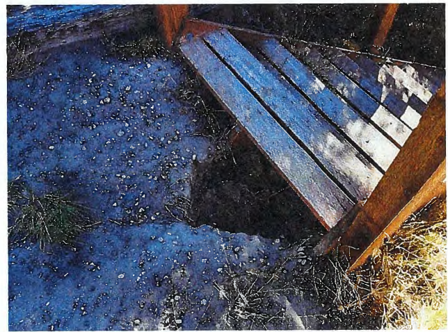
Figure 2: Erosion gullies can be seen extending from parking lot elevation down to the water surface; additional damage is visible below ordinary high water.
