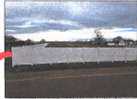
6ft White vinyl fencing to fully surround staging area
