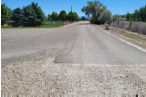
Stoffle Lane – public section of road
